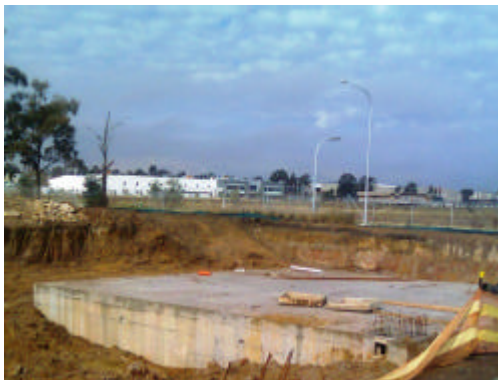
800 kL stormwater tank under construction
